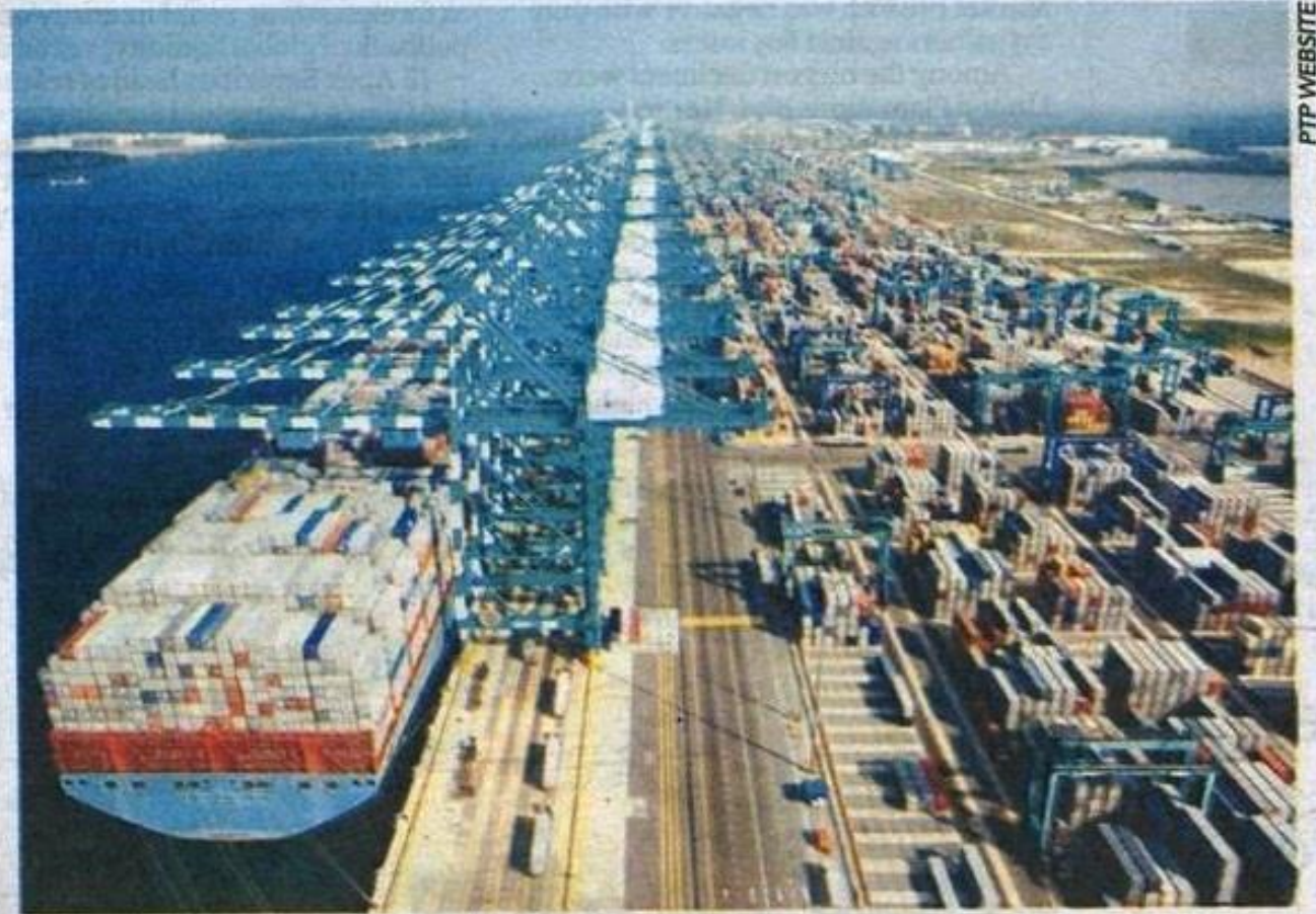
Container vessels loading and unloading at Port of Tanjung Pelepas.
