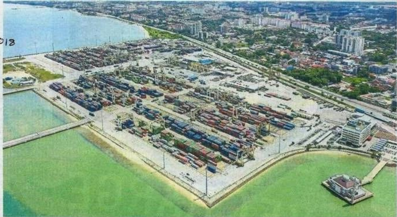
Revamp underway: An aerial view of NBCT in Butterworth, Penang.
